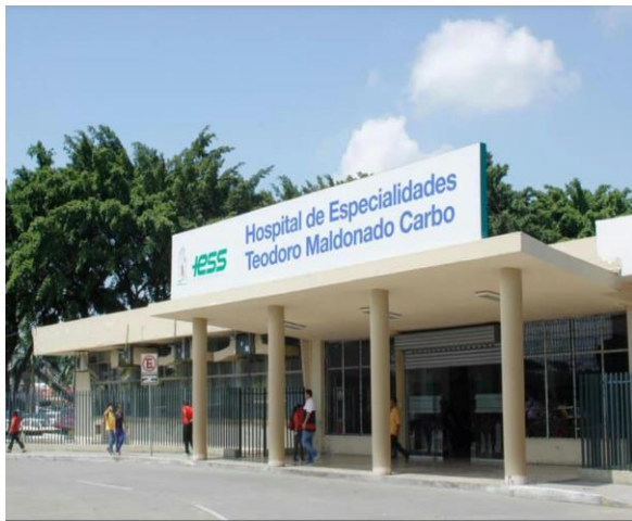
Fachada del Hospital TMC
